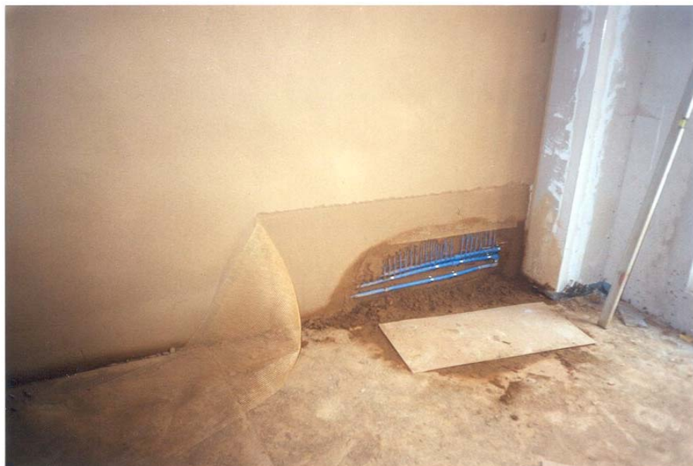
Picture 2: Earthen plaster on a wall-heating-system
